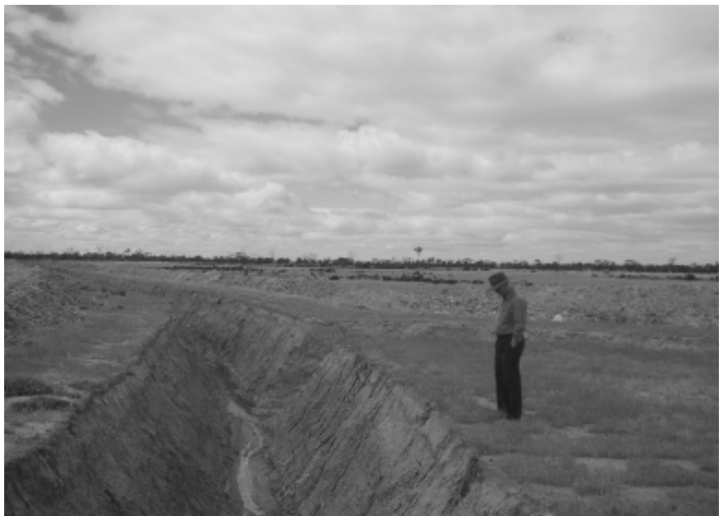
Photograph 3.2 Deep drainage systems being trialled at Dumbleyung, Western Australia
