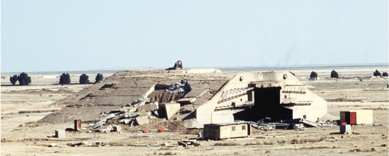
Figure 32: Hardened Aircraft Shelters (HAS) require considerable effort to defeat, often needing multiple bunker busting bombs. Smaller smart bombs and cruise missiles are typically unable to penetrate effectively (US DoD).
