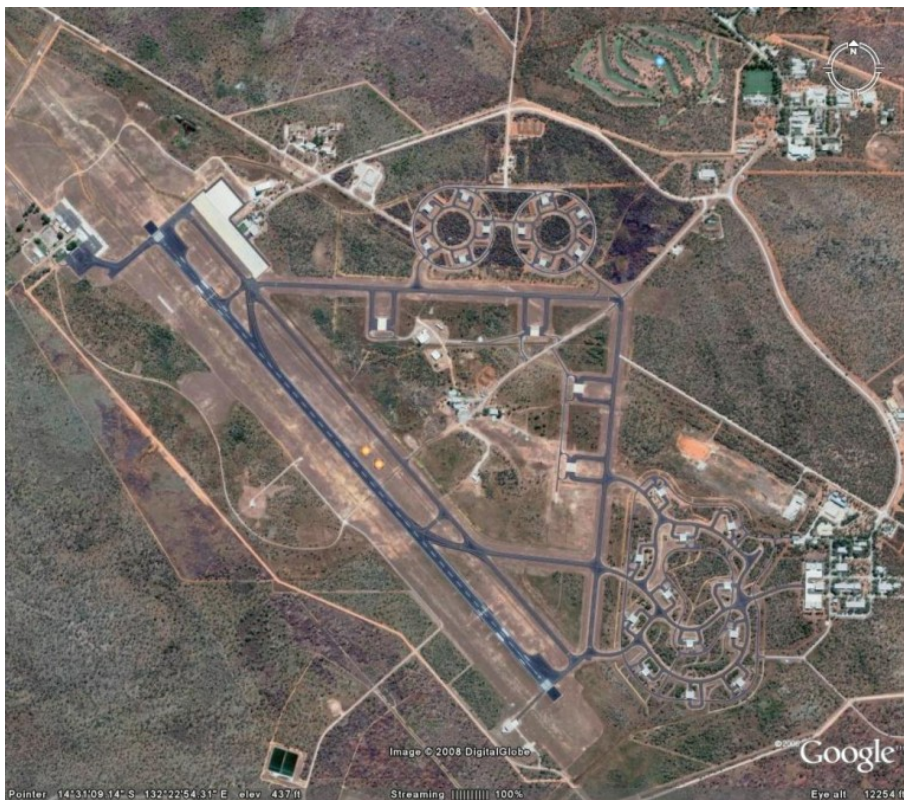
Figure 33: The absence of proper base hardening measures, especially Hardened Aircraft Shelters (HAS), presents a major strategic vulnerability in this era of widely available cruise missiles and smart bombs. Depicted the strategically vital RAAF Learmonth and Tindal sites (Google Earth).
