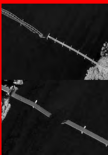
DESTRUCTION OF TRANSPORTATION INFRASTRUCTURE
