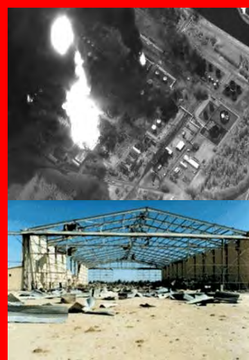
DESTRUCTION OF ENERGY INFRASTRUCTURE AND INDUSTRIAL PLANT
