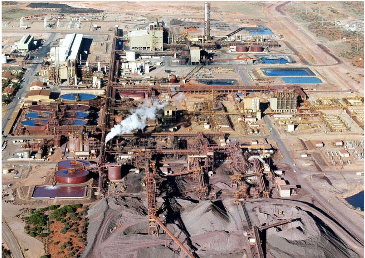
Figure 3.7 Processing facilities at Olympic Dam in South Australia
