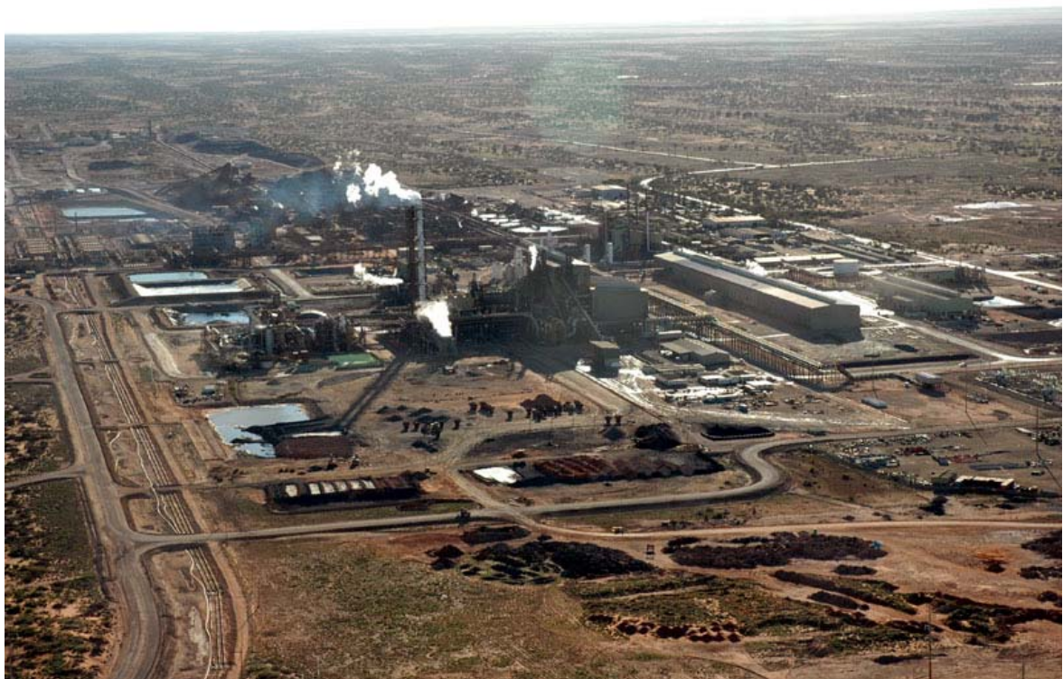
Figure 3.8 Aerial view of Olympic Dam
