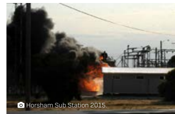
Horsham Sub Station 2015.
