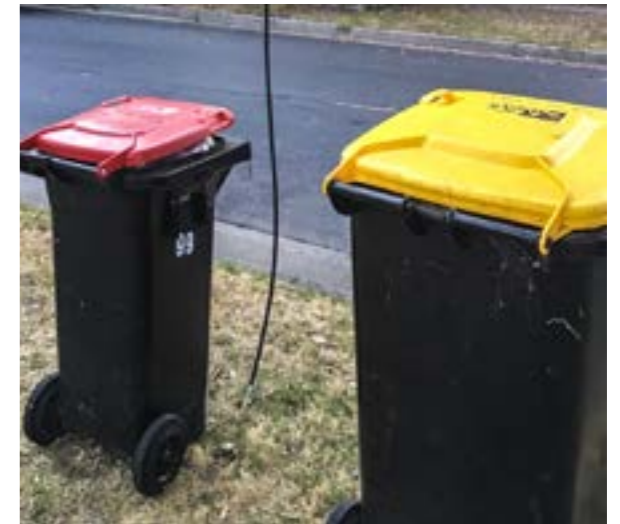
📍 A recent example of a live service wire in suburban Melbourne that failed due to age and deterioration. Reports from residents stated the wire had hung alive opposite a sports ground for 2 days before crews responded.
