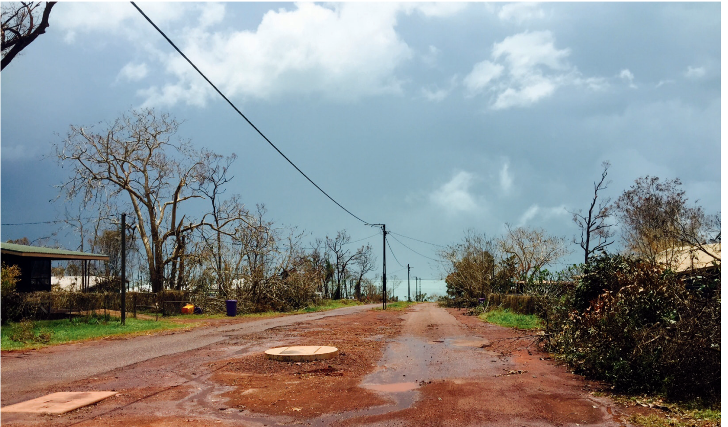
Cyclone Lam damage, Galiwin'ku, Elcho Island, NT, 2015 ( Australian Red Cross )
