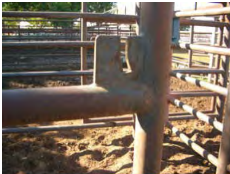
A chain hitch on a swing gate. This is the most secure slot design.
