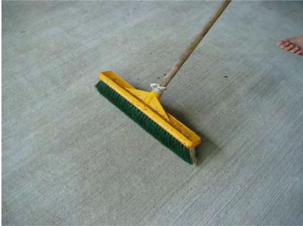
Surface on concrete described as broom finish. A broom finish will give a good non-slip surface for cattle. Brush strokes to be at 90° to the direction of the movement of cattle.
