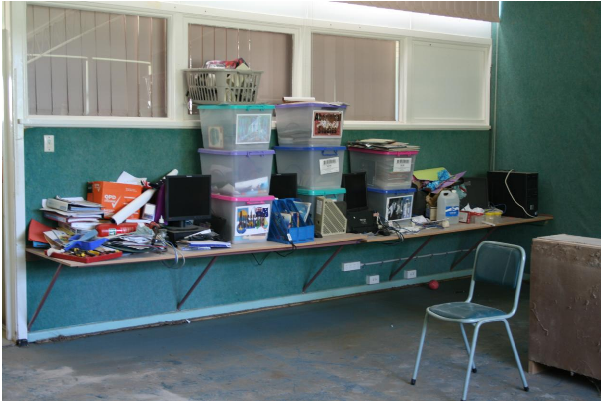
The computer bench in the Senior Classroom. These benches are not designed for weight bearing yet heavy resource boxes were stacked on top and in between valuable computers. The bench is now damaged.
