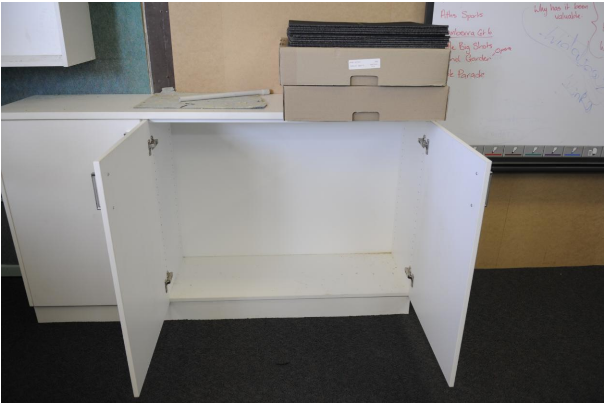
The new joinery was installed in the Senior Classroom but without shelving which made it difficult to reinstate classroom resources.
