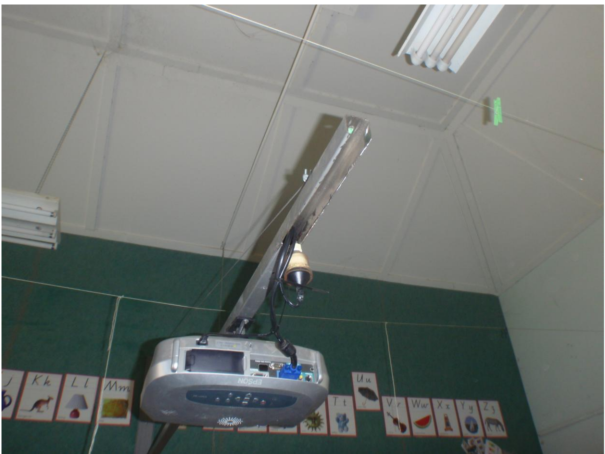
The raw edge of the projector arm which, as of 14 th of May, is still in this condition.
