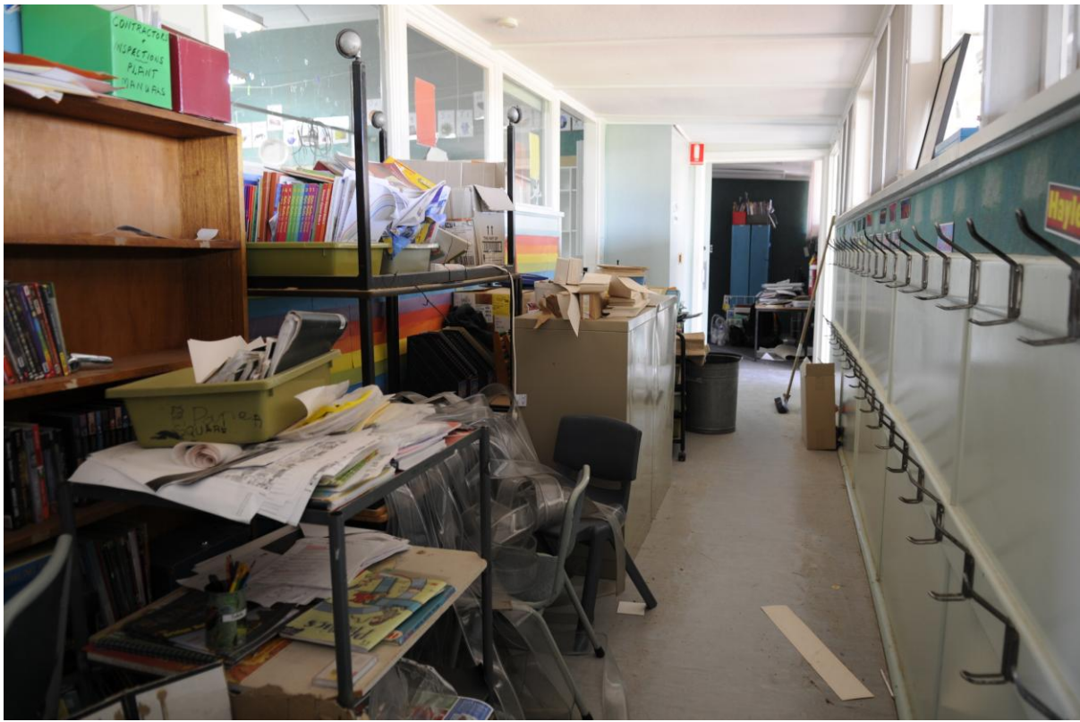
The school corridor, leading to the library and kitchen/staff room.
