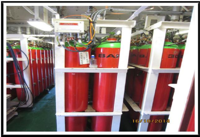
It is unclear how the LR Surveyor could make a visual examination of all cylinders from outside the room given the arrangement of the cylinders as depicted in the above photo.
