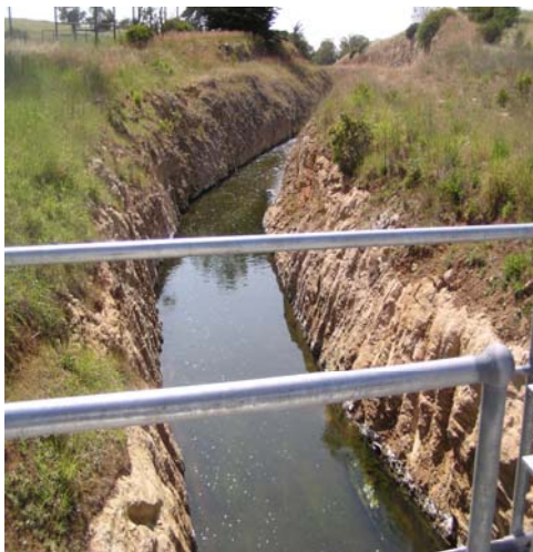
South East Drain (SA) (photo: L Burge)
