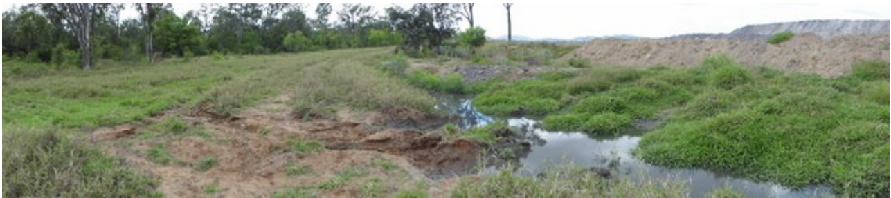
Coral Creek Sonoma 12.9.10 – 11am . Signs of levee bank channel overflow.
