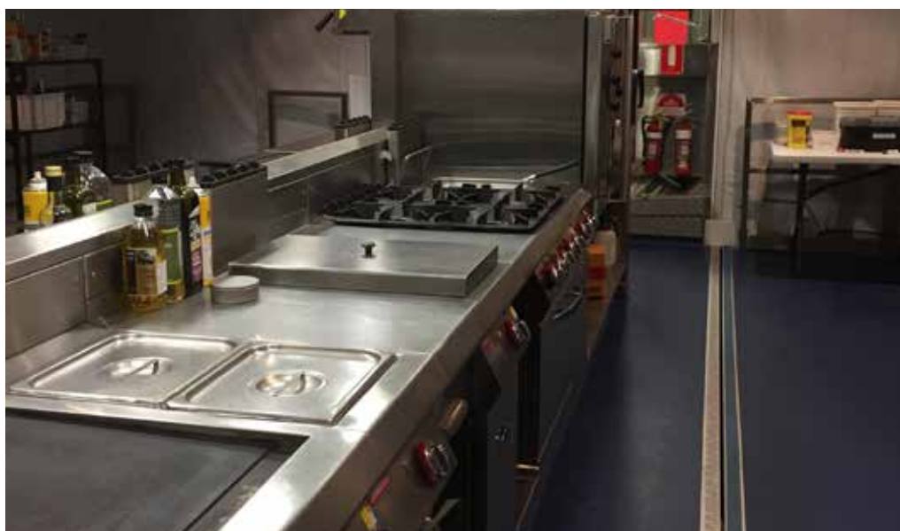
Equipment in the 'Big Red Truck.'
