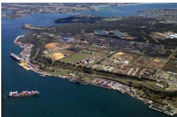
Bell Bay Port Tasmania
