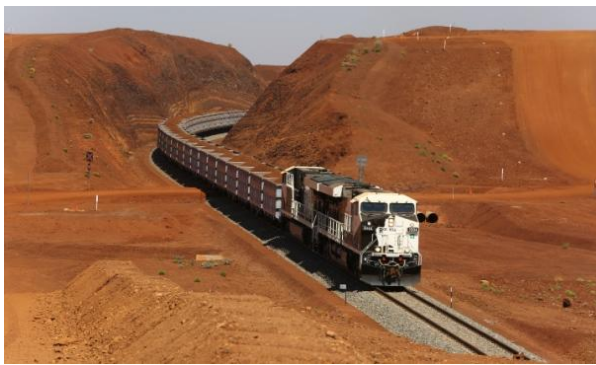
Figure 2: Pilbara long haul freight rail - world's best practice
