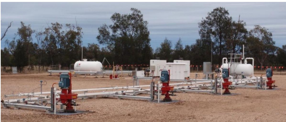
Below: Four well pad in Pickanjinie in Fairview Field, Queensland
