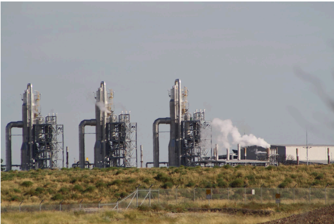
Emissions from reverse osmosis plant, photo courtesy of local resident
