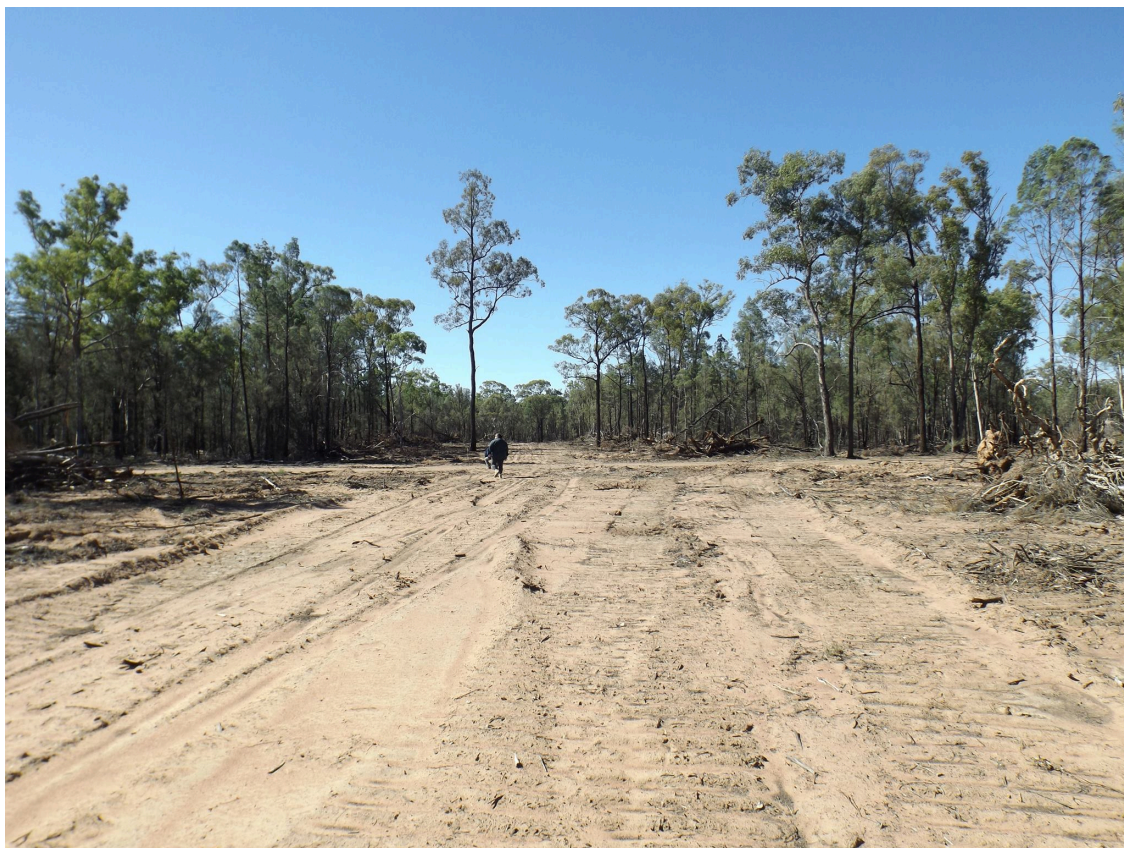
Environmental impact, massive bulldozed 'laneways' criss-cross the site, photo courtesy of local resident
