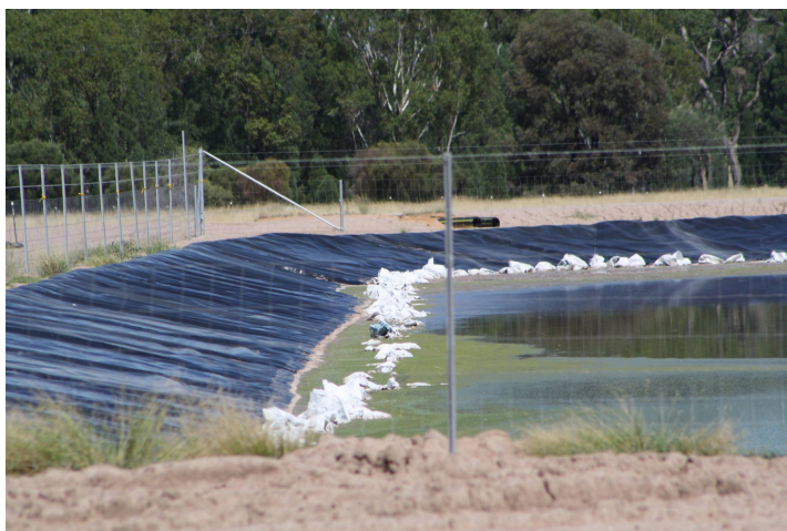
Open sewage pit, photo courtesy of local resident
