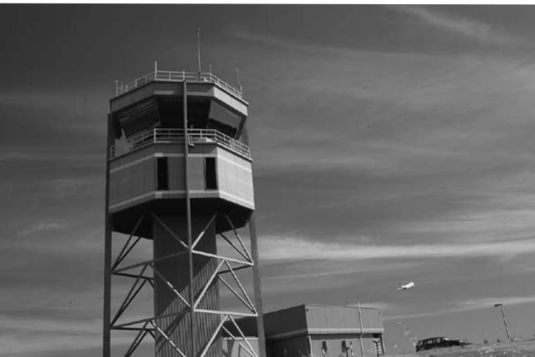
Below: Adelaide air traffic control tower.
