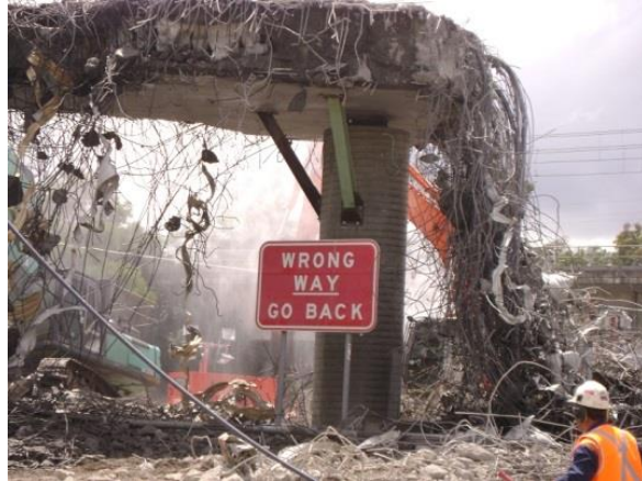
Right: bus ramp pulled down
