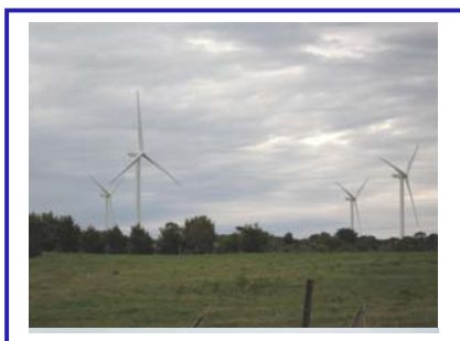
View of turbines at Wonthaggi wind farm
