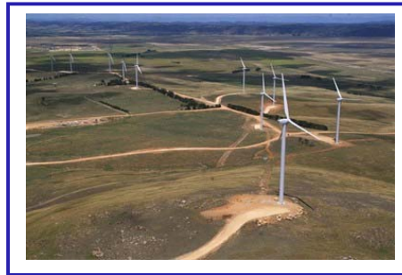
View of turbines at Capital wind farm
