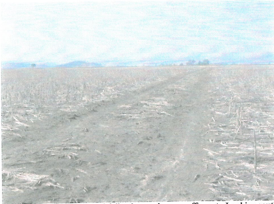
Erosion damage to the crown road following a minor runoff event. Looking south from junction of Crown and Public Road. February 2009
