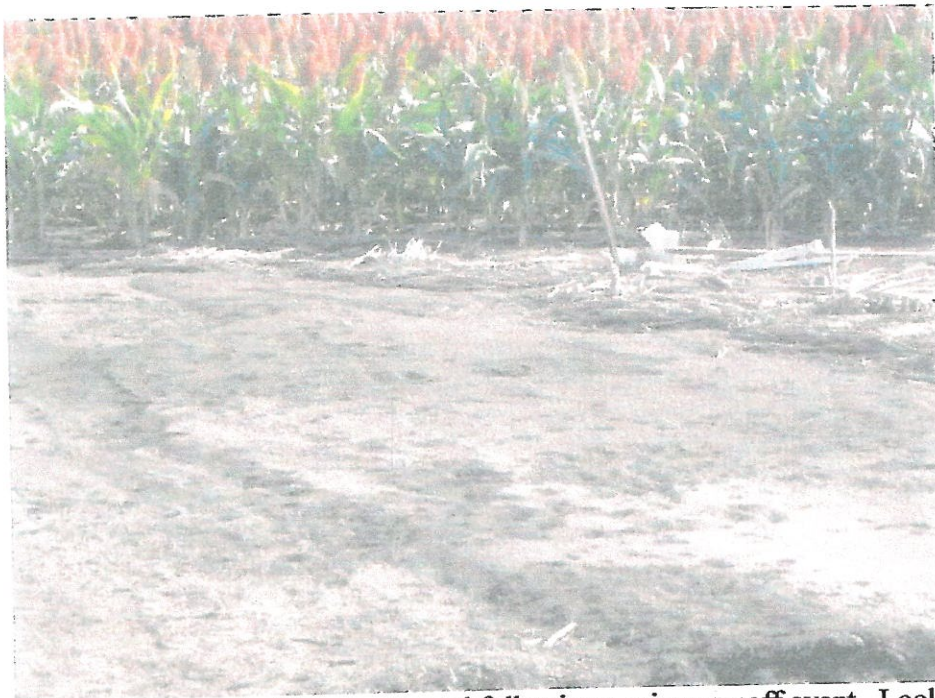
Siltation at the northern end of the crown road following a minor runoff event. Looking north at the junction of Crown and Public Road. February 2009
