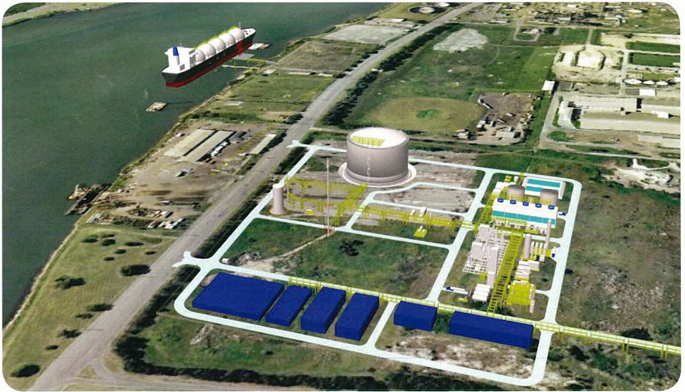
Schematic of LNG Newcastle Project at Kooragang Island (Image courtesy of Toyo Engineering Corporation)
