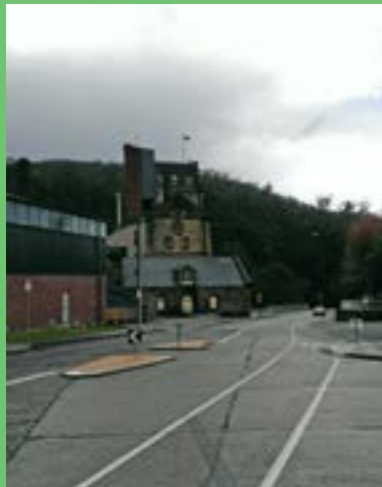
Hobart City Council has installed a pedestrian refuge on Strickland Ave at Cascade Brewery and included an uphill bike lane as part of the project. This short link provides a connection for bicycle riders using the Hobart Rivulet path from the Cascade Gardens to the Old Farm Road turnoff.
