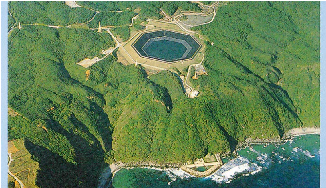
Figure 6 Pilot Seawater Pumped-storage Power Plant, Okinawa Pref. in Japan. The octagonal shape shows the upper dam. The outlet of the tailrace is surrounded by tetra-pods for protection from waves. The picture is from the 1998 Hitachi Review.
