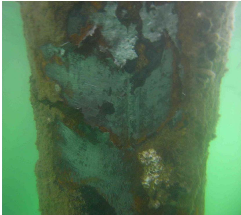
Photo 2 - Pile detailing exposed concrete
