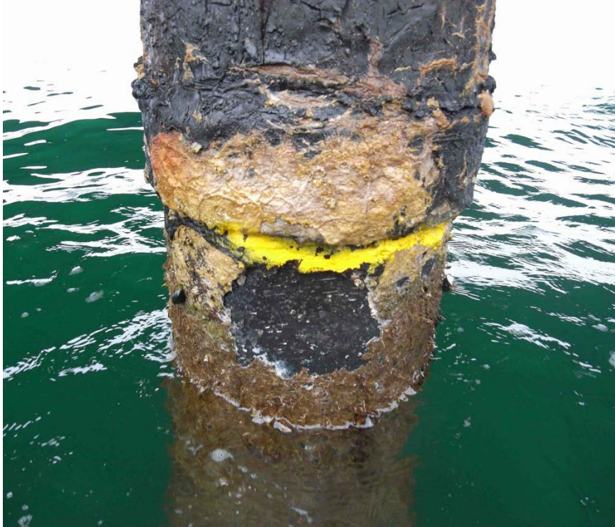
Photo 1 - General Condition of Piles
