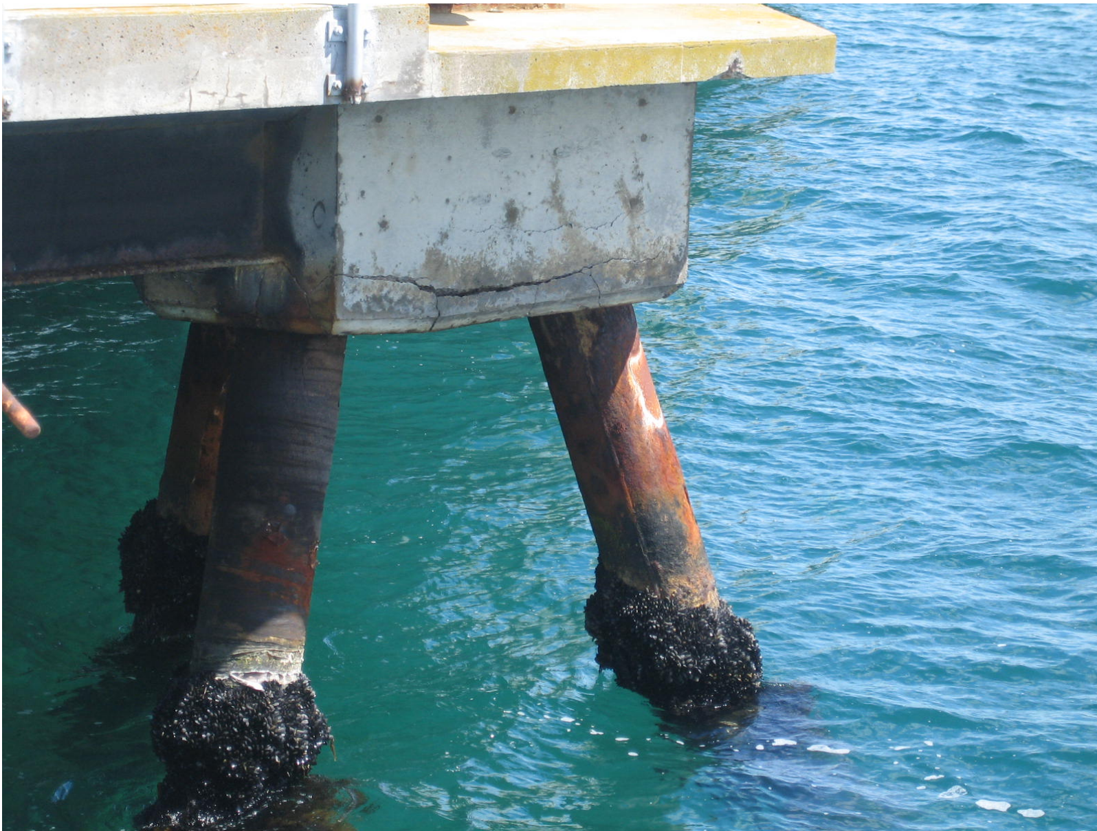
Photo 4 - General Condition of Wharf
