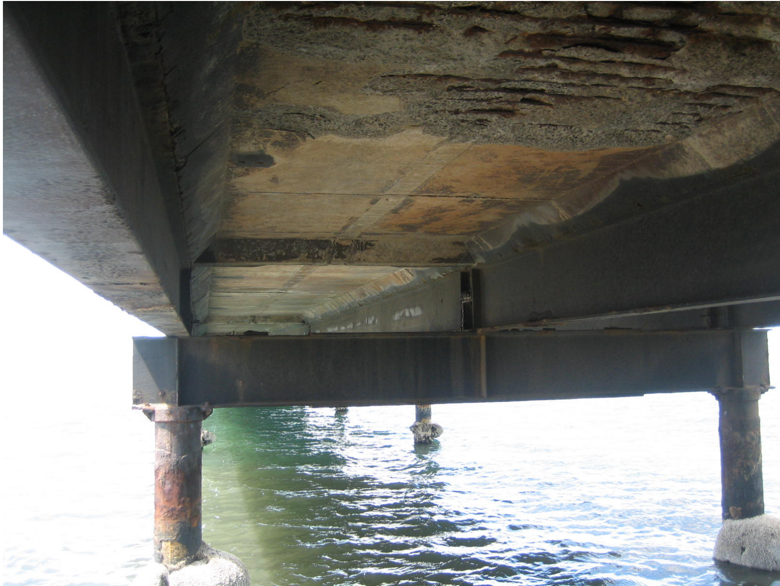
Photo 3 - General Condition of Piles, Crossheads and Jetty
