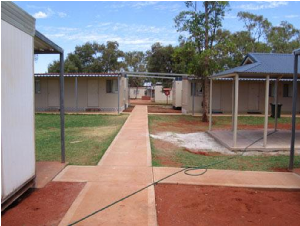
Accommodation blocks, Leonora alternative place of detention, November 2010.
