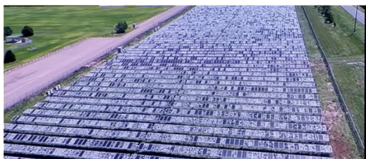
Hail-damaged solar cells for landfill
