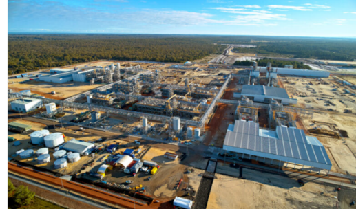
Aerial view of WA's Kemerton Li(OH) plant. Image: Albemarle.
