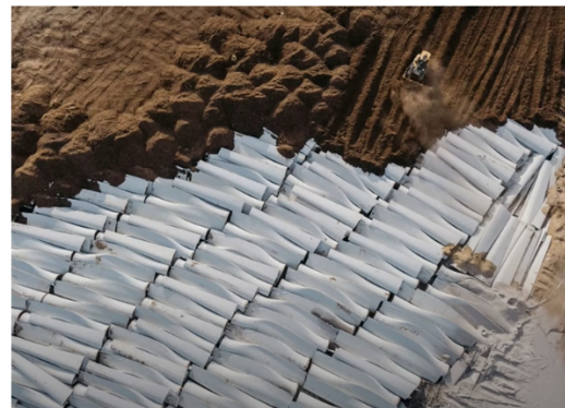
January 9, 2020: wind turbine blades being buried in the Casper WY Regional Landfill.
