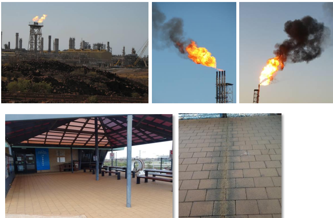
Figure 5. Emissions from the Woodside industrial plant on Burrup Peninsula (above), photograph of Woodside Visitors Centre showing small gap between two roof lines (lower left) and degradation of paving bricks where rain falls between the two roofs, with the dark colour suspected to be from microbial growth adjacent to the erosion line (lower right).
