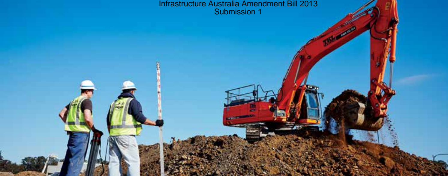
Hunter Expressway, NSW
