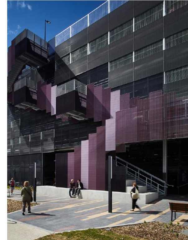
Dawson Street car park, Sunshine
