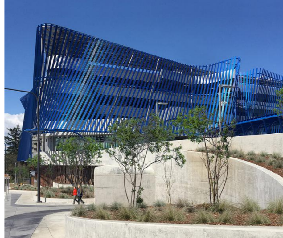
Angle Lake car park, Seattle
