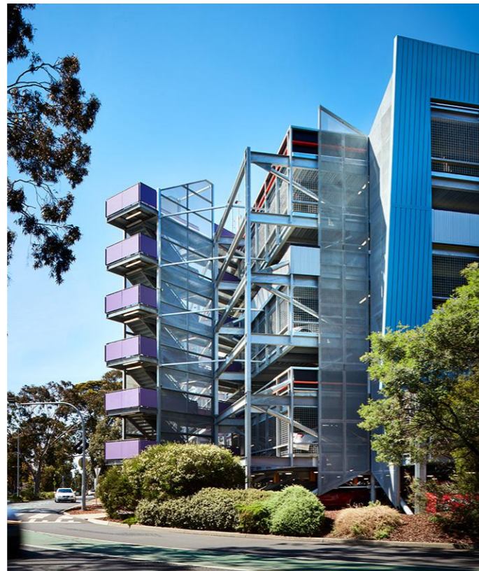
Monash University car park, Clayton
