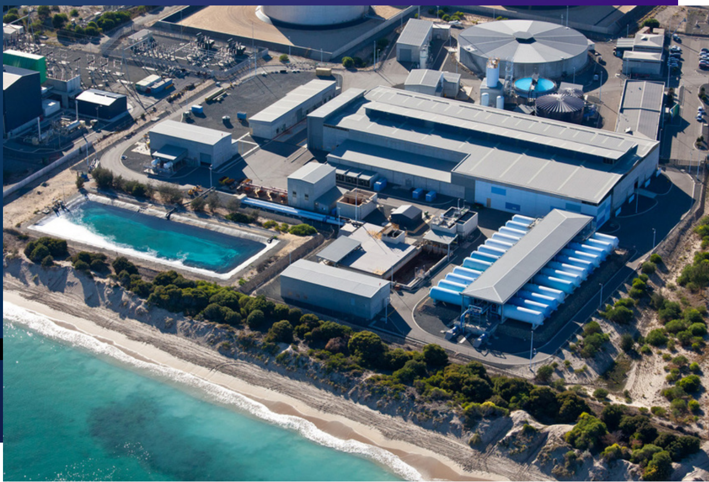
Perth reverse osmosis desalination plant
