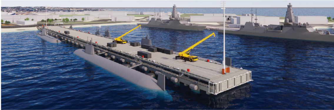
Artist's impression of HMAS Stirling Main Base Precinct – Project Element 1 maritime infrastructure. Upgraded berthing infrastructure and dredging for nuclear-powered submarines.
