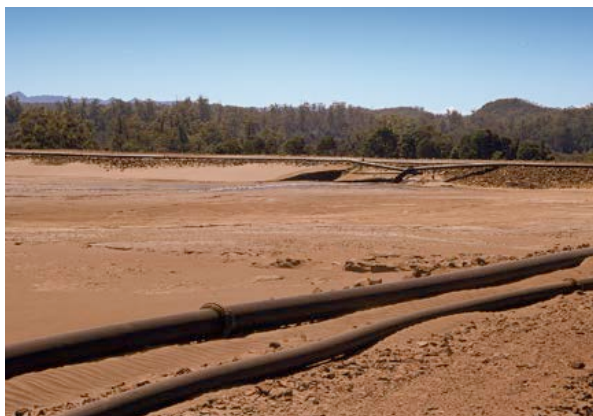
The cassiterite flotation tailing cover across the tailings at the start of the TSF rehabilitation in 1992.
