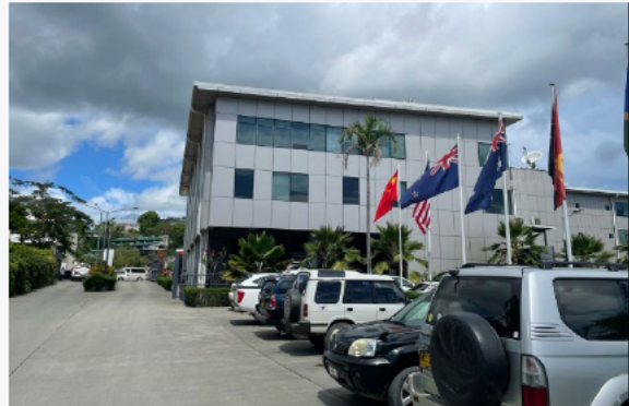
Street view looking at building outside
