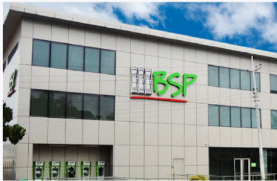
Street view looking at building outside
