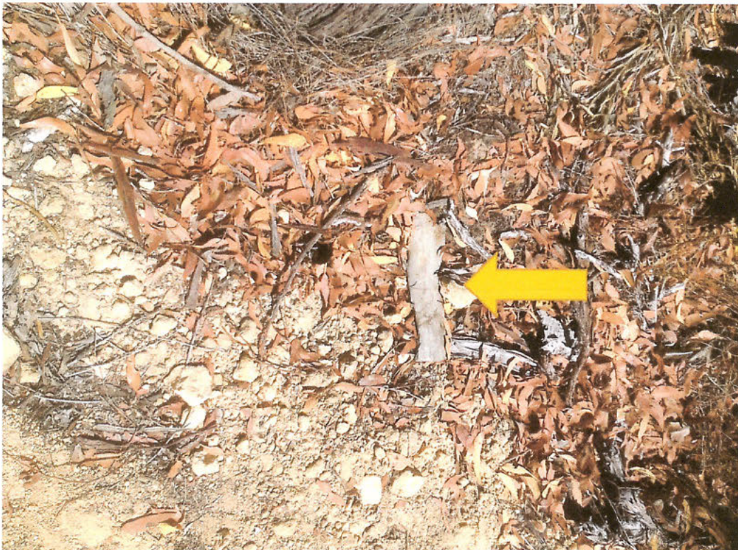
Asbestos piece inside the fenced area after the alleged clean-up of asbestos.
