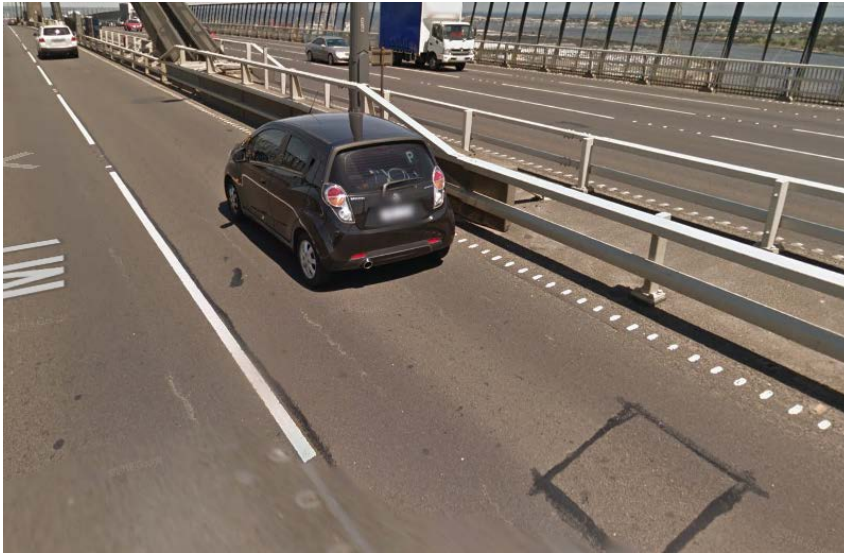
Figure 36: West Gate Bridge Edge Line and Barrier (Source: Google Maps)
