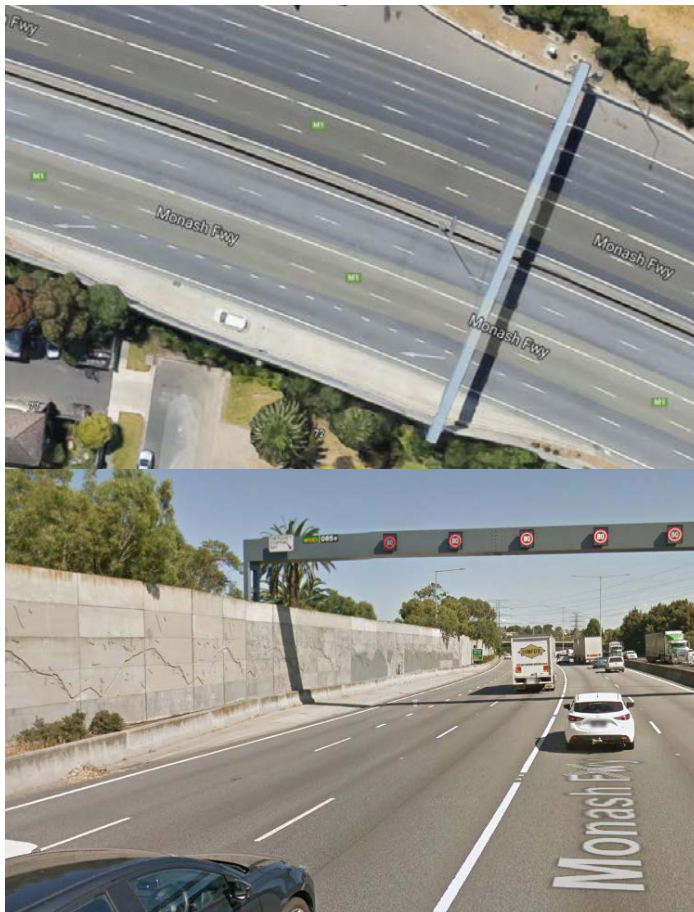
Figure 40: Monash Freeway - Emergency Bay (Source: Google Maps)
