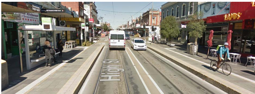
Figure 32: High St, Northcote - Tram Stop
