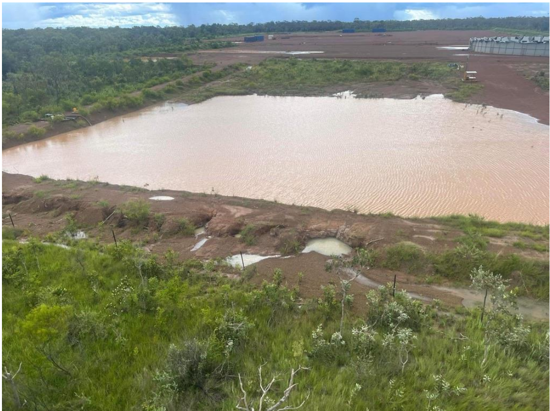
Courtesy Protect Big Rivers 4 Bund wall giving way on Maverick well pad, known site of contamination.
