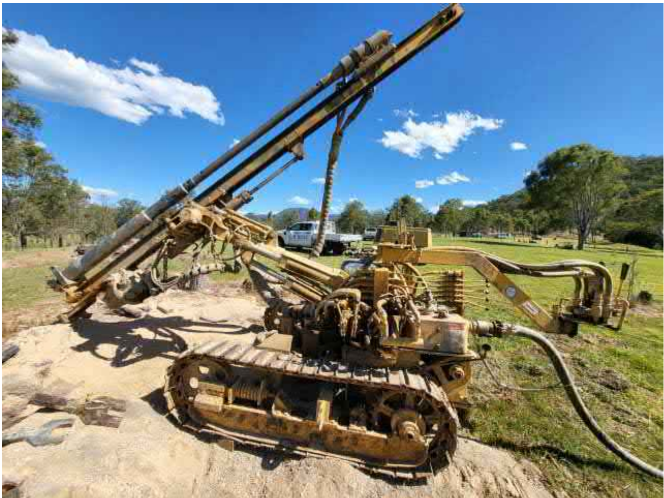
Figure 4.1 Measured rock drilling unit
