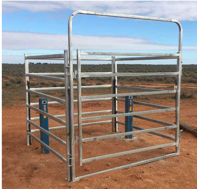
Figure 31 Bore headworks completion at W02S and W02C
