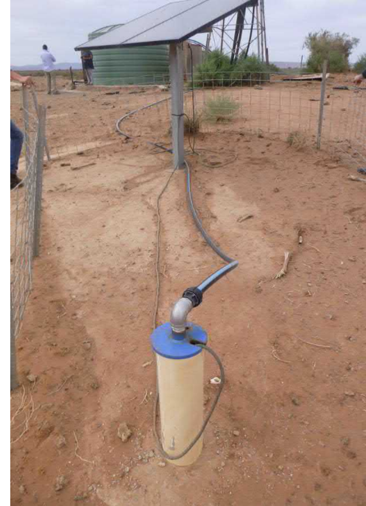
Well 6534-360 pump, power and tank set up.
