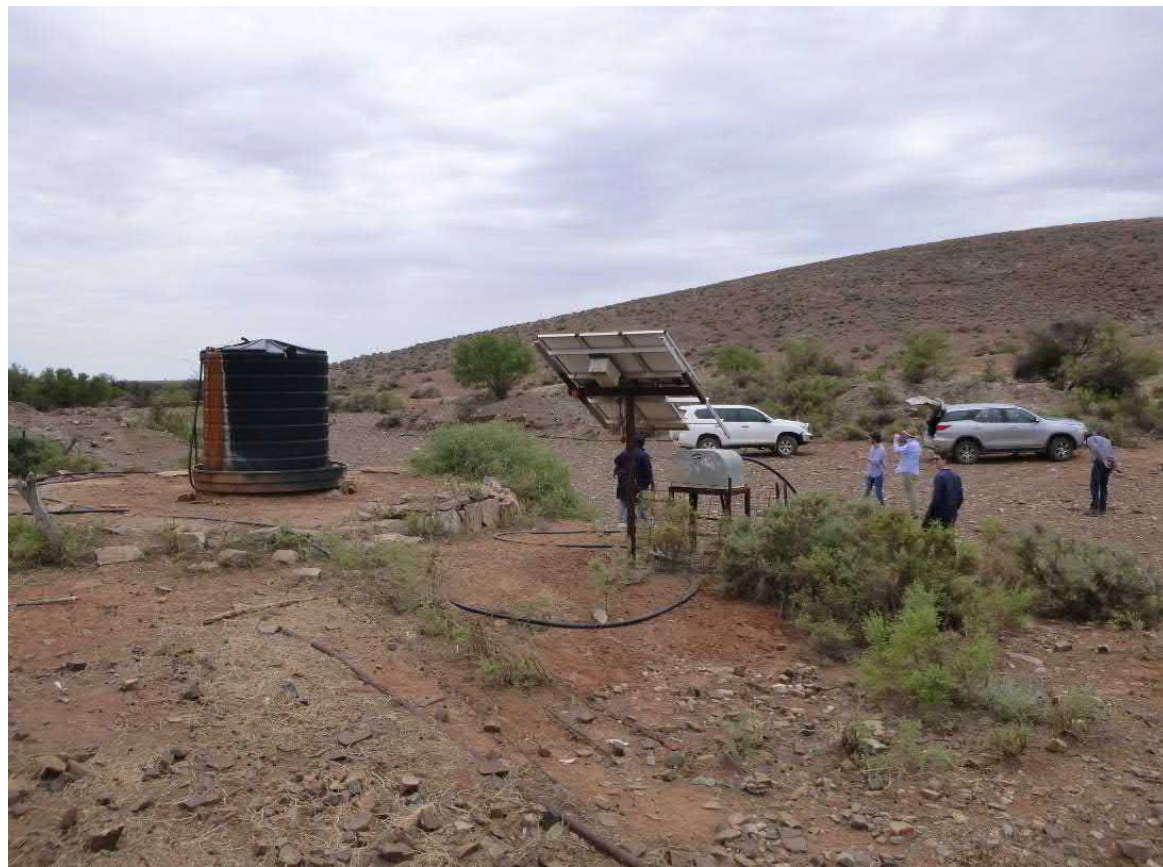
Close up of Murrays Bore set up. Water level was measured at 1.6 m below top of casing, total well depth was 39 m below top of casing on 21/02/18.
