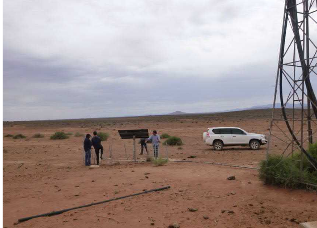
Well 6534-360 (East Yallala Bore) replacing 6534-25, solar pump relaces windmill for stock water.
