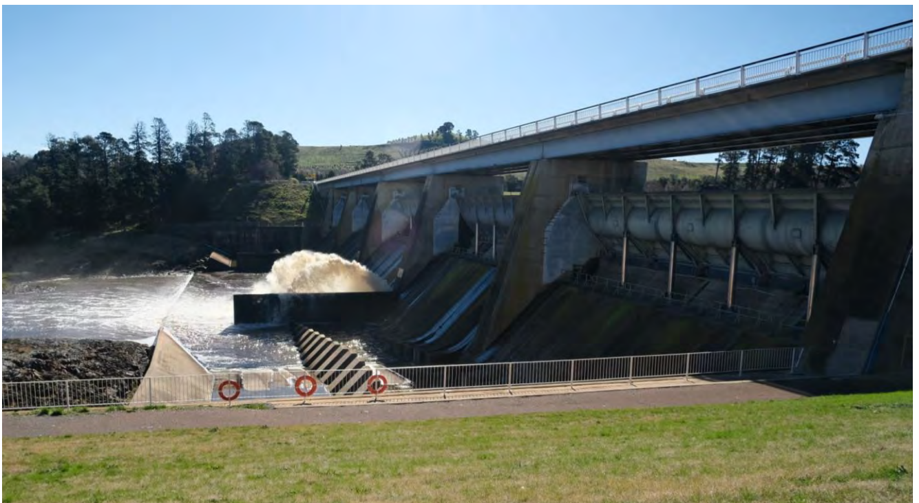
Figure 4 Photo of Scrivener Dam from left abutment
