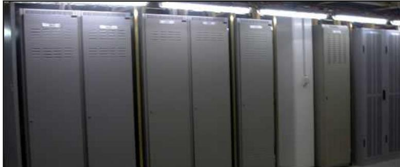
This (above) is a typical installation of several racks<sup>16</sup> of (iiNet) DSLAM equipment all in physical competition with Telstra, Optus and other DSLAM equipment, all in the one in a (Telstra) metropolitan exchange site, and separate Points of Interconnect.
