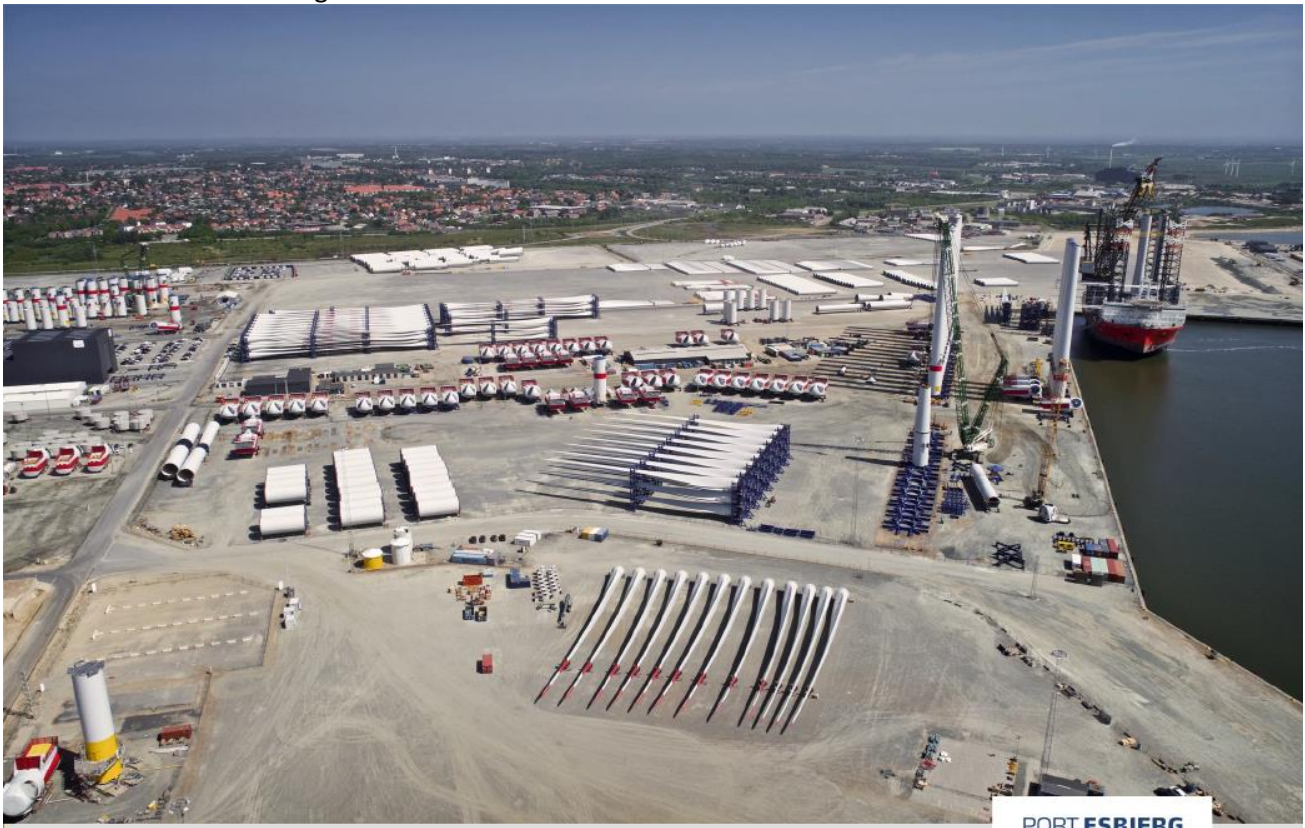
Figure 2: Part of the Port of Esbjerg, Denmark, which handles vast quantities of components for onshore and offshore renewable energy. There are multiple wind turbine component manufacturing and assembly facilities in the surrounding area.
