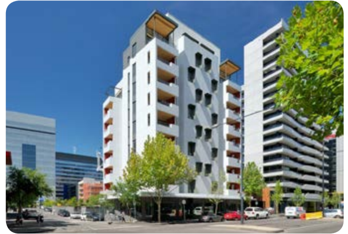
Figure 7.3: Forte building – 10-storey apartment block, Docklands, Melbourne
