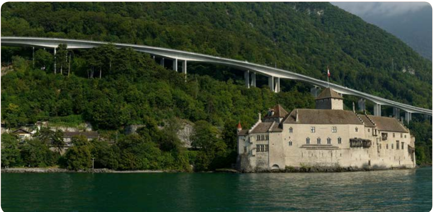
Figure 7.1: The Chillon viaducts which connect France and Switzerland were upgraded using ultra-high strength concrete (Ductal). Photo credit: Hartmut Mühlberg
