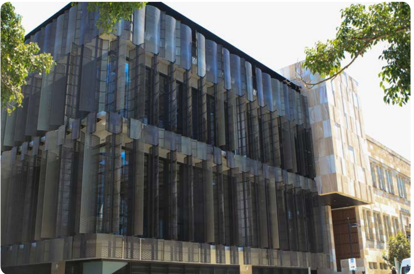
Figure 4.8: Global Change Institute, University of Queensland made from Wagners' Earth Friendly Concrete
