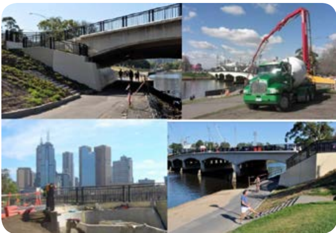
Figure 4.5: Retaining walls made from Zeobond's E-Crete at Swan St Bridge, Melbourne
