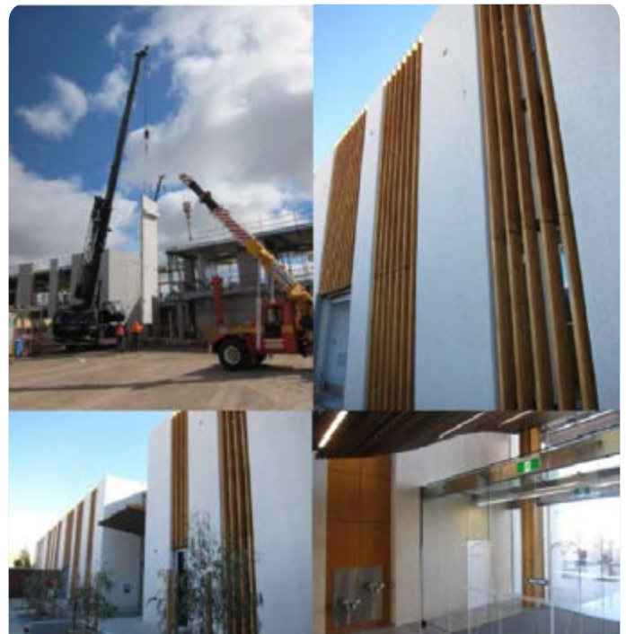
Figure 4.7: E-Crete precast panels at Melton Library
