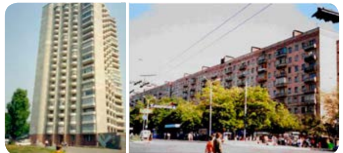
Figure 4.1: (left) 20-storey residential geopolymer concrete building, Lipetsk, Russian Federation, 1987–1989; (right) 9-storey geopolymer residential buildings, Mariupol, Ukraine, 1960 48
