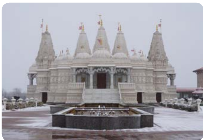
Figure 5.2: BAPS Shri Swaminarayan Mandir, Chicago. Foundation slab made with 65% fly ash cement.
