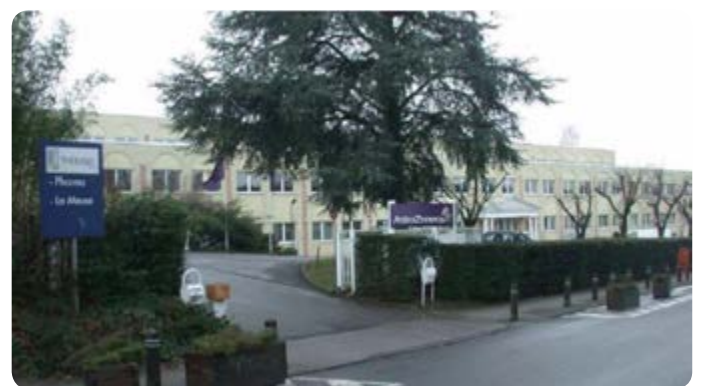
Figure 4.2: Les ateliers Delle in Ukkel, Belgium built using a geopolymer called Purdocement in 1957
