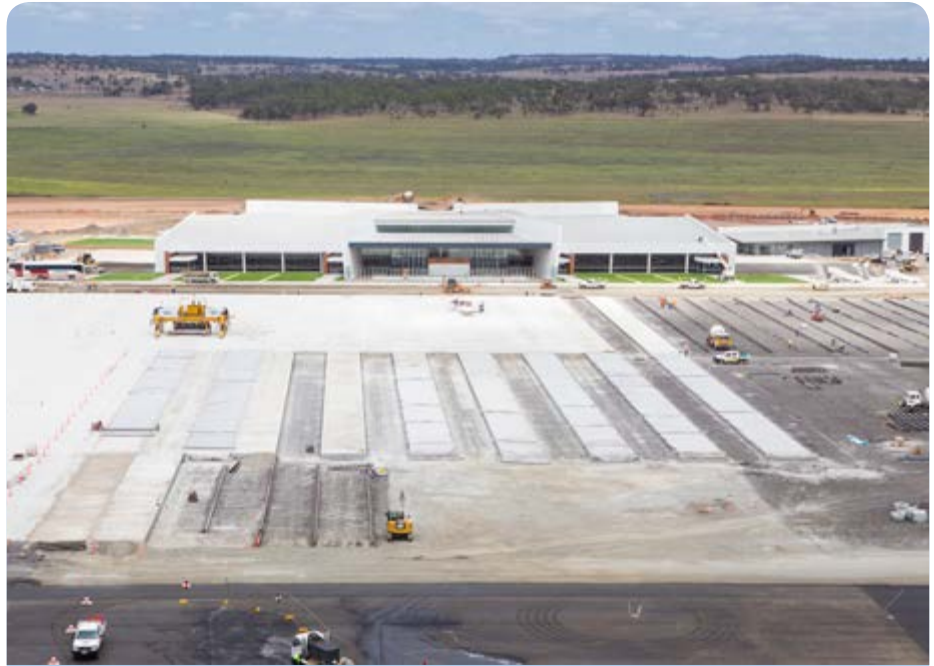
Figure 4.9: Brisbane West Wellcamp Airport
