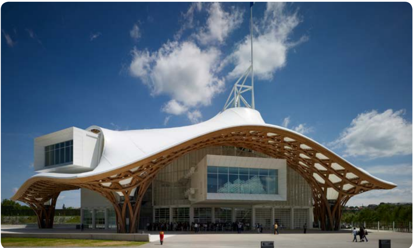
Figure 7.2: Timber roof of Centre Pompidou in Metz (Photographer: Didier Boy de La Tour)
