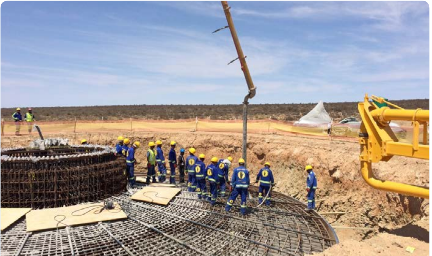
Figure 5.1: Loeriesfontein Wind Farm – turbine foundation
