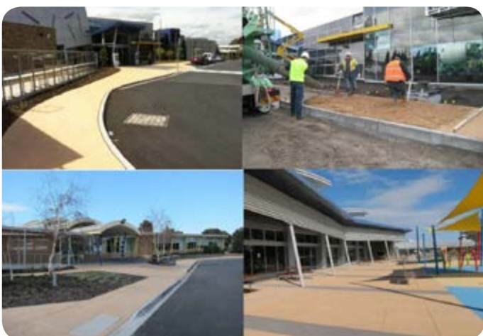
Figure 4.6: Pavement made from Zeobond's E-Crete at Thomastown Recreation and Aquatic Centre.
