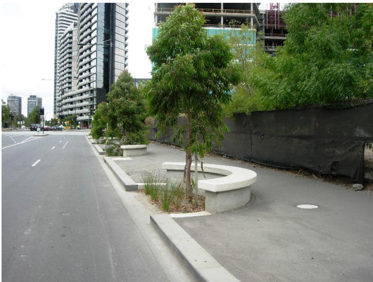
Figure 42: Batman Drive bioretention tree pits, Docklands Melbourne. By author.
