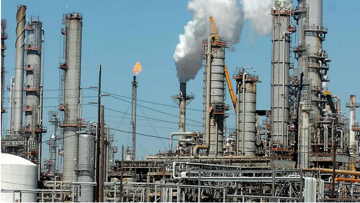
Ethylene Cracker https://www.sofisglobal.com/securing-safe-ethylene-production-use-valve-interlocks
