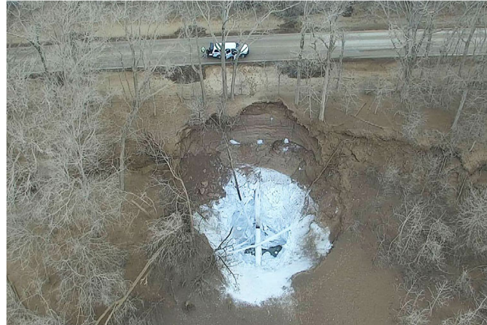
A carbon dioxide pipeline rupture in Mississippi sent at least 45 people to hospital in 2020 https://www.eenews.net/articles/biden-releases-plan-to-avoid-dangerous-co2-pipeline-failures/
