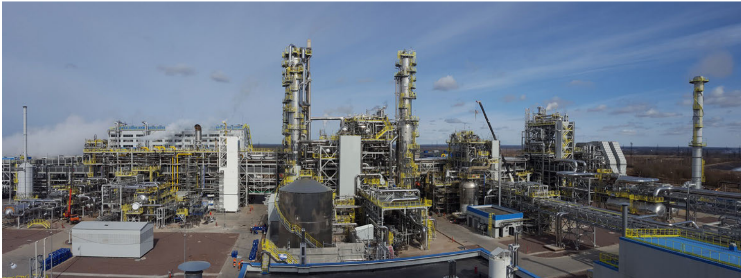
Ammonia Plant Russia https://www.tecnimont.it/en/what-we-do/fertilizers/kingisepp-ammonia-production-plant
