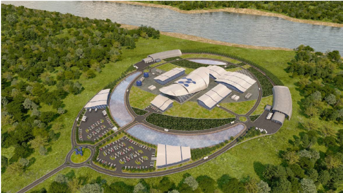
Image: NuScale Power SMR, 12 x 77 MWe modules, 924 MWe total on an 13 hectare site. US Nuclear Regulatory Commission (NRC) Final Safety Evaluation Report issued in August 2020 - first SMR to achieve NRC design approval.
