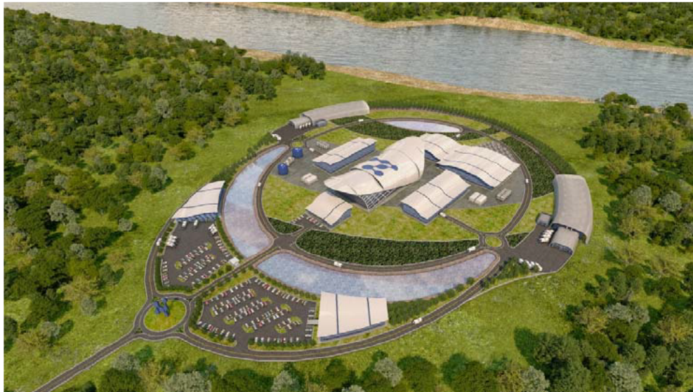
Image: NuScale Power SMR, 12 x 77 MWe modules, 924 MWe total on an 18 hectare site.
