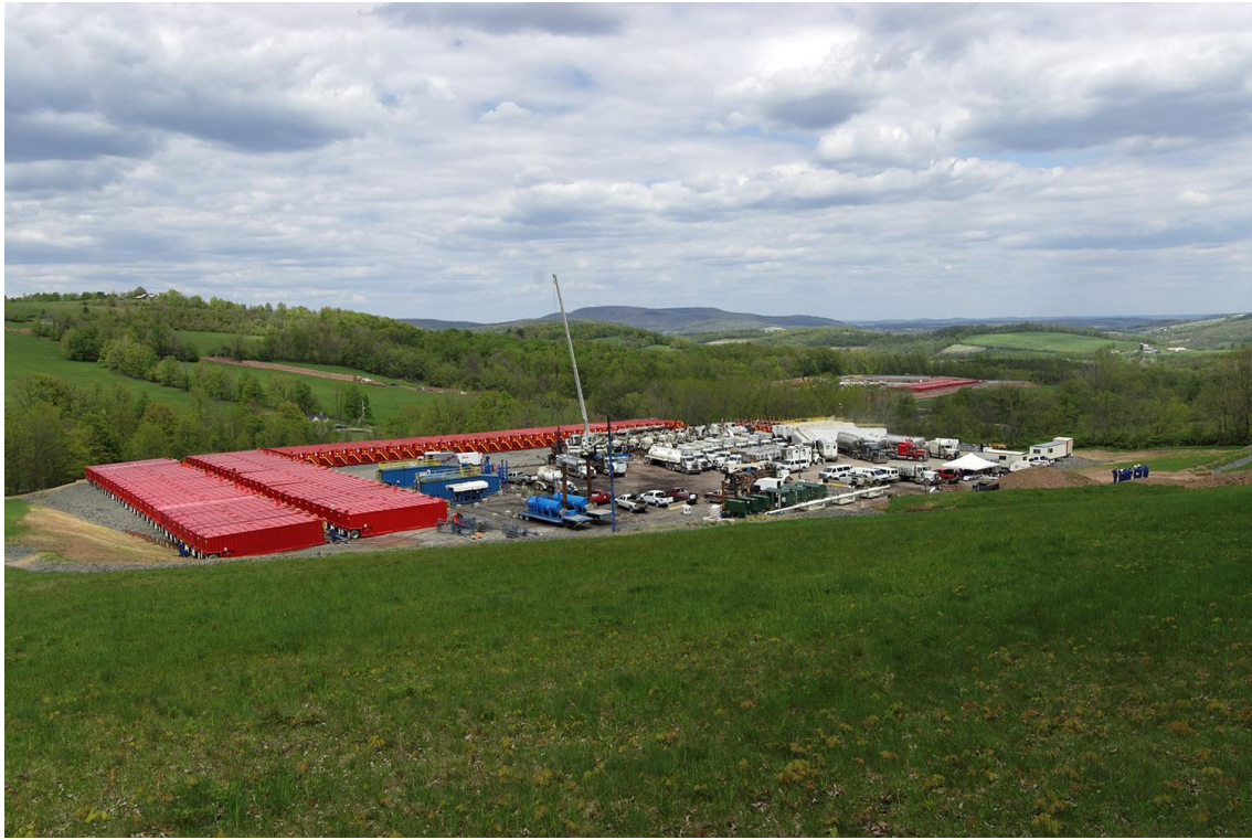
Photo 6.5 - A representative view of active high-volume hydraulic fracturing (New August 2011)
