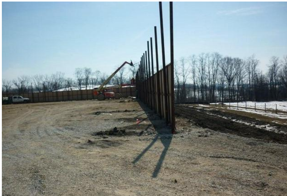
Photo 7.4 - Sound Barrier Installation (New August 2011)
