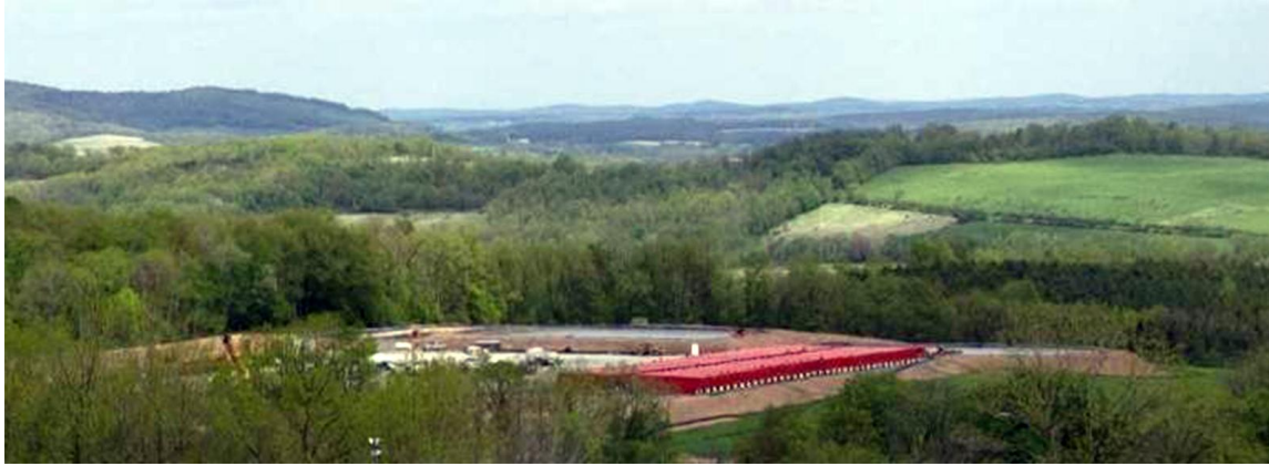
Photo 6.3 - A representative view of a newly constructed water impoundment area (New August 2011)
