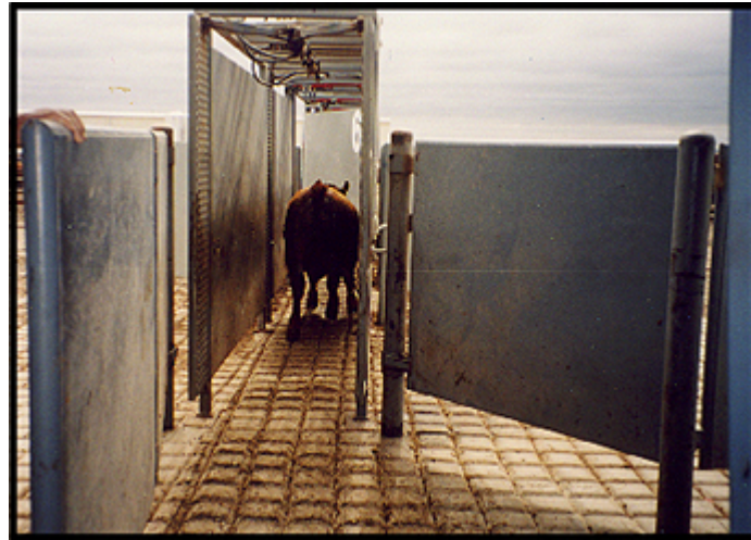
Figure 3. Deep square pattern for handling facilities for beef cattle. The squares are 20 cm (8 in) by 20 cm (8 in). The V shaped grooves are a minimum of 2.5 cm (1 in) deep and 2.5 cm (1 in) wide. The grooves can be made by pressing angle iron into the wet concrete or making a stamp. Pour a practice slab first to learn how to do it. The pattern can not be properly made if the concrete starts to set. Do not use this pattern in dairies. It will be too rough for cattle to walk on every day. It is intended for use in handling facilities such as truck loading ramps, feedlot handling facilities, stockyards, slaughter plants, and other places where cattle occasionally walk. These grooves can also be made in a diamond pattern that will make washing easier. Orient the points of the diamonds towards the drain.
