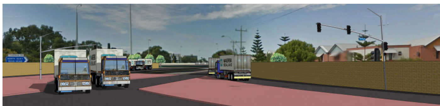
Figure 18. A before and after shot of the intersection of Tydeman and Stirling in North Fremantle. High sounds walls and wide turning radii allow 80 km per hour truck movements with light priority through this narrow urban area.
