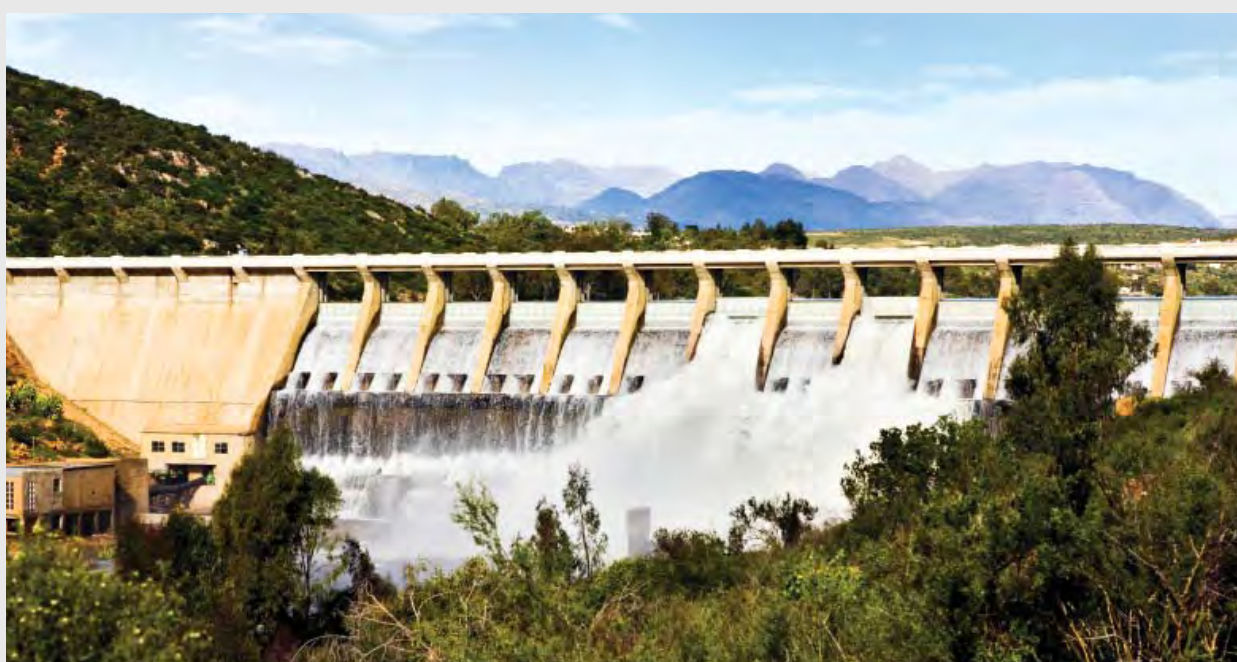
Figure 3. Dam sluiceways are an example of graceful degradation and seamless reintegration of a system under stress.
