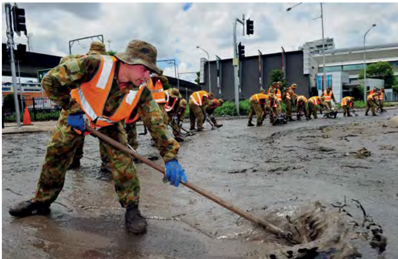
Figure 36: Soldiers in the Australian Army clear mud and sludge from a major intersection in Queensland after extensive flooding.
