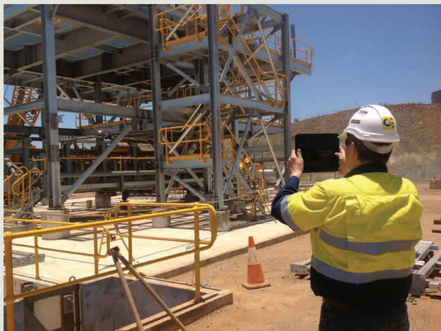
Use of a tablet computer onsite allows the project team to view the project's 3D model, as well as access work packs (library of 2D, 3D and specification information), construction check sheets, and defects and issues reporting.
