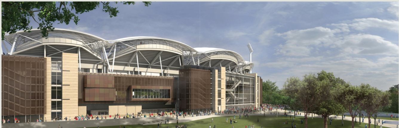
To develop the Adelaide Oval, multiple team members from a variety of disciplines needed to author and access project data. The team created a BIM execution plan to contractually establish terms and expectations.
